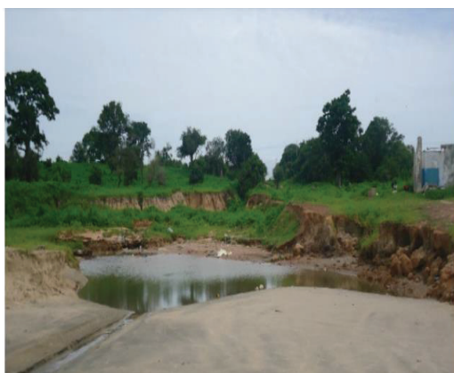
(v) Coastal Erosion along Kololi
