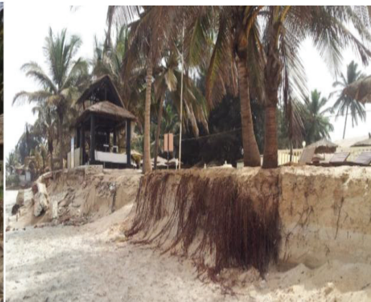
(iv) A Structure at Risk Due to Coastal Erosion
