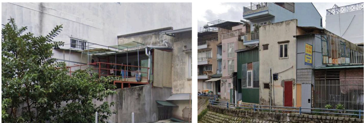
Fig. 6: Current functional use of caged balconies at housing along To Ngoc Van Canal
