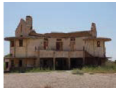
10: Bovardeh neighborhood-2floors– at the same time with the start of Abadan Oil Company and Refinery
