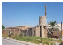
6: Ziba bathroom · 1934, closed
