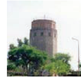
8: North Bovardeh Water Reservoir, Obsolete
