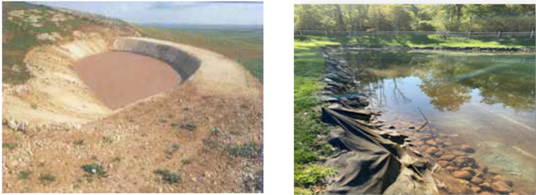
Fig. 7: showing types of water pan/ pond with a) local water pan, b) retention ponds (Mati, 2012)
