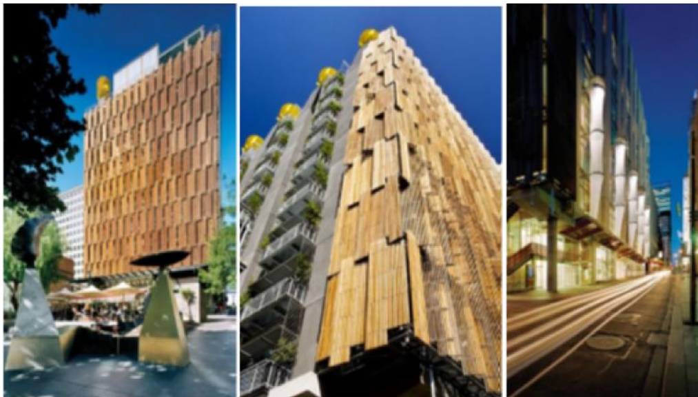
Fig. 1: CH 2 building: right: spray of water to cool the southern facade, middle: A view of the exhaust flue (North), left: Western view (Pearce, 2014)
