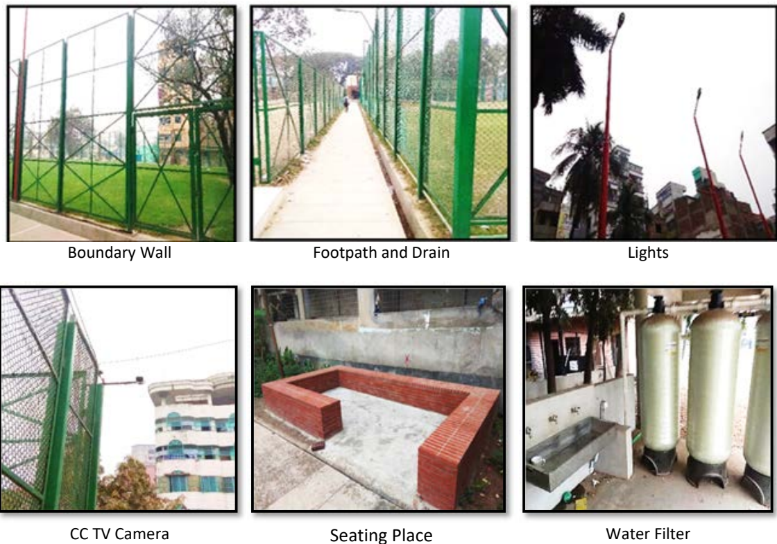
Fig. 4: Newly Installed Infrastructure
