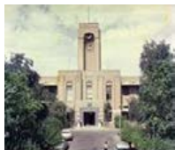
9: The Petroleum University, 1939, Still working
