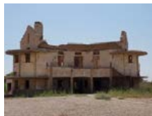
10: Bovardeh neighborhood-2floors– at the same time with the start of Abadan Oil Company and Refinery
