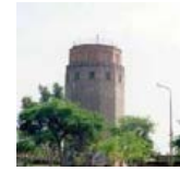
8: North Bovardeh Water Reservoir, Obsolete
