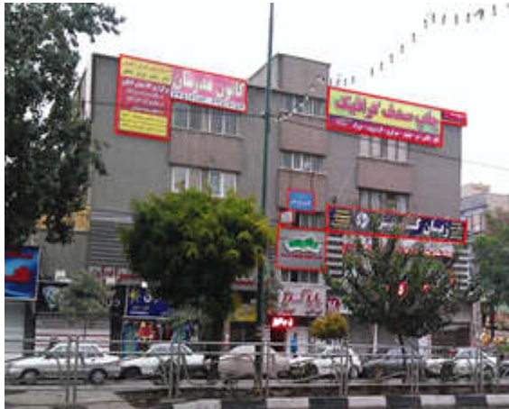
Fig. 7: Installing the inappropriate billboards on the façades; Golshahr District, Karaj
