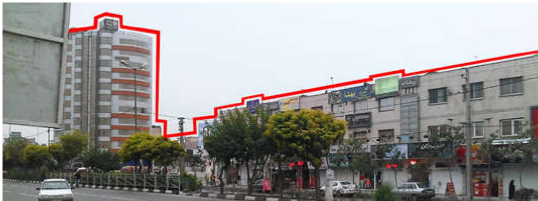
Fig.6: The deterioration of the skyline due to the lack of balance in the building heights and densities; Golshahr District, Karaj
