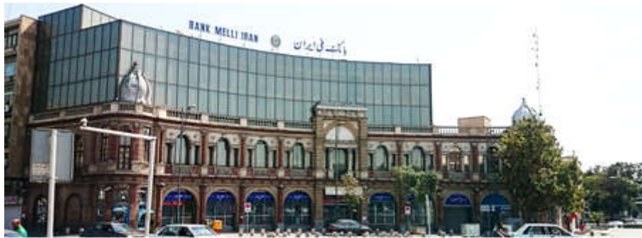
Fig. 1: The revival of a historical façade within one of the sides of Hassan Abad Square in Tehran. This façade has currently been regenerated over the modern building which had been built during the Pahlavi period. This action has obviously strengthened the physical identity of the existing historical façade and also the surrounding urban environment
