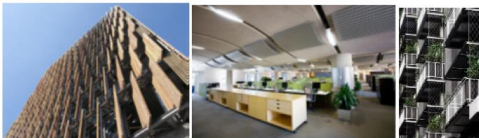
Fig. 6: the interior space of the building: right: the northern terraces - middle: office units - left: windows used for ventilation (Meinhold, 2009)
