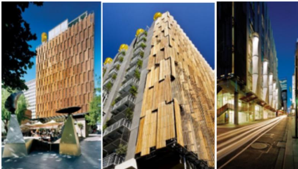
Fig. 1: CH 2 building: right: spray of water to cool the southern facade, middle: A view of the exhaust flue (North), left: Western view (Pearce, 2014)
