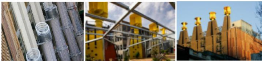
Fig. 5: CH 2 building: right: northern view (air suction ducts) - middle: the roof structure – left: light-colored vents on the southern façade (Meinhold, 2009; Pearce, 2014).
